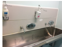
Taps designed to reduce the risk of cross contamination
